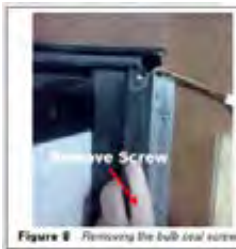
Figure 8 Removing the bulb seal screw
